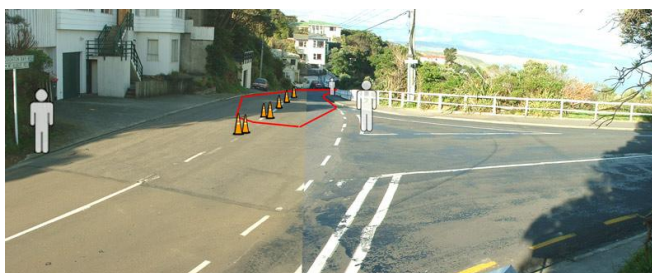
Buckley Road turn viewed from just past the turn point
